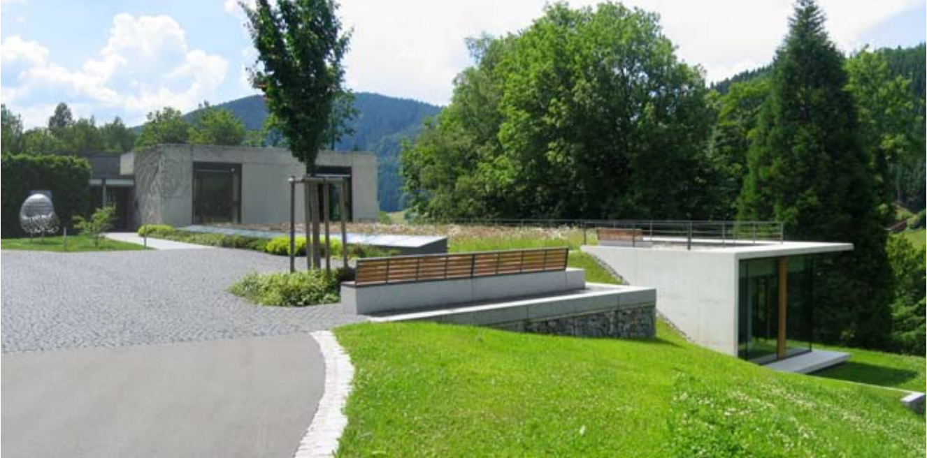
View of the new part of the building and entrance area
