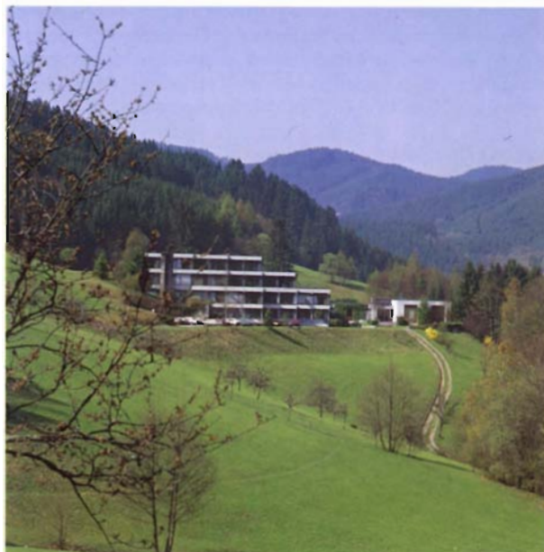
View from the North-East, in the foreground: the guest-house bottom: the staggered building with library and discussionrooms from the South
