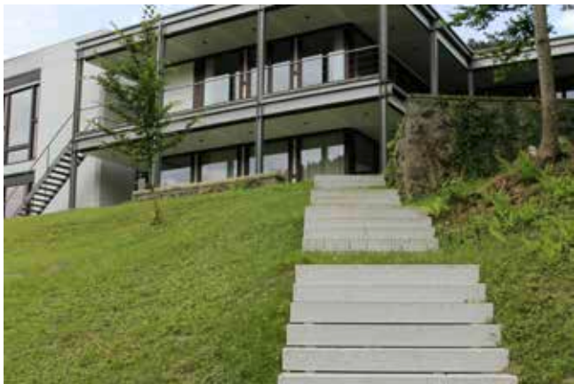
Treppe an der Bibliothek / Staircase at the library
