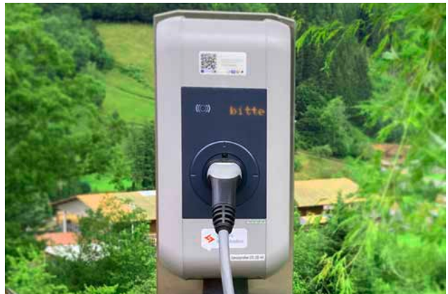
Ladestation für E-Autos / Charging station for electric cars
